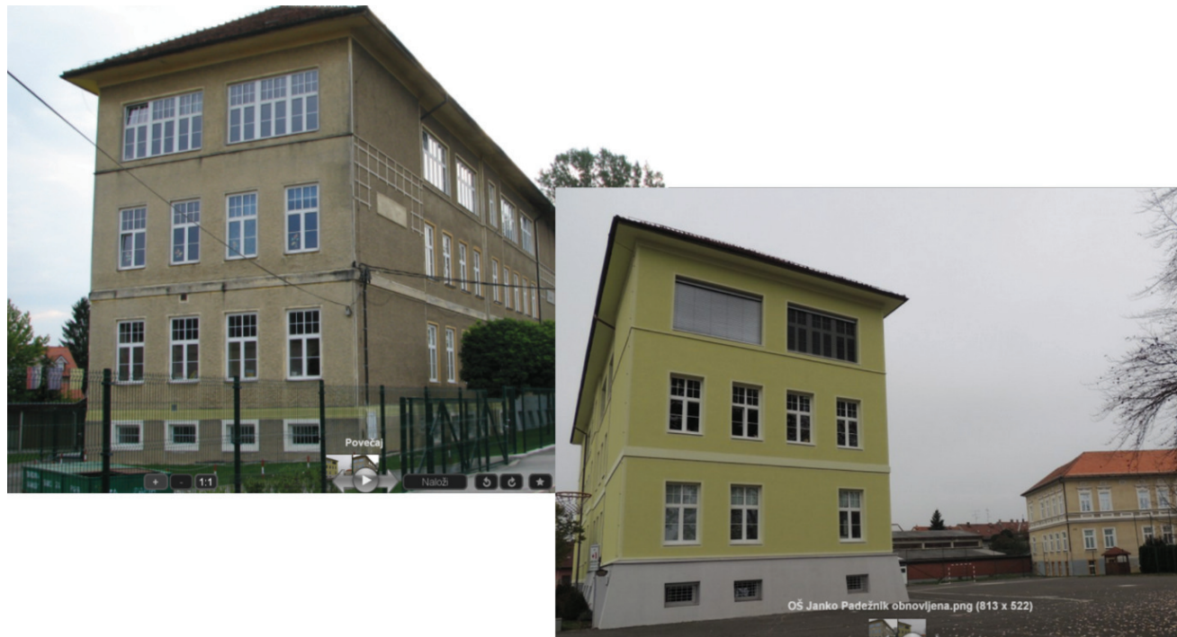
One of the 24 renovated public buildings in the municipality Maribor (primary school)
